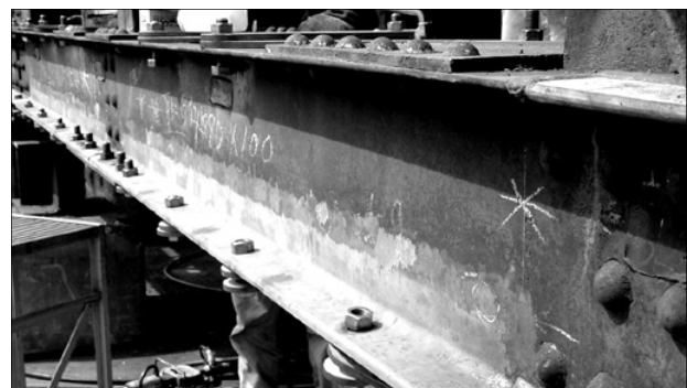
図4 下弦材の補修状況 Repair of chord members
