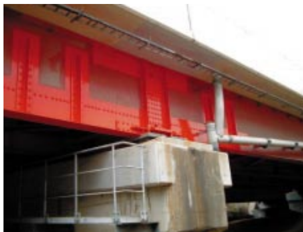
図8 桁連続化工法 Girder-connected continuous bridge system
