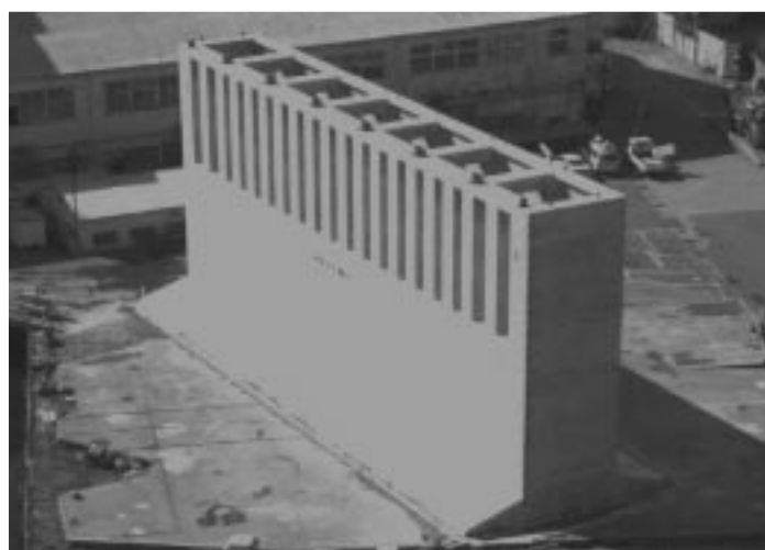
横須賀港大津地区防波堤 Breakwater in Yokosuka Port Otsu District
