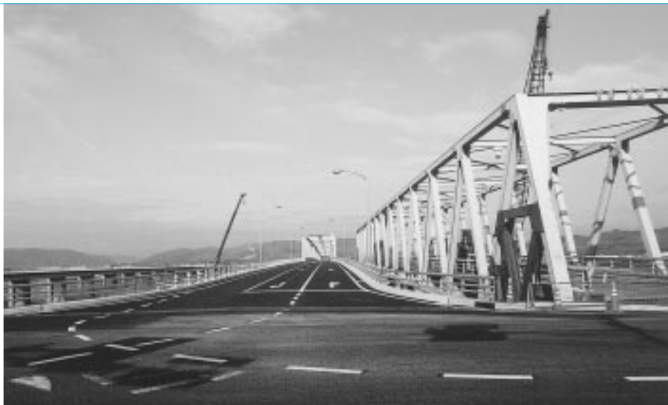
図1 川辺橋架替え Kawabe-bashi Bridge replacement
