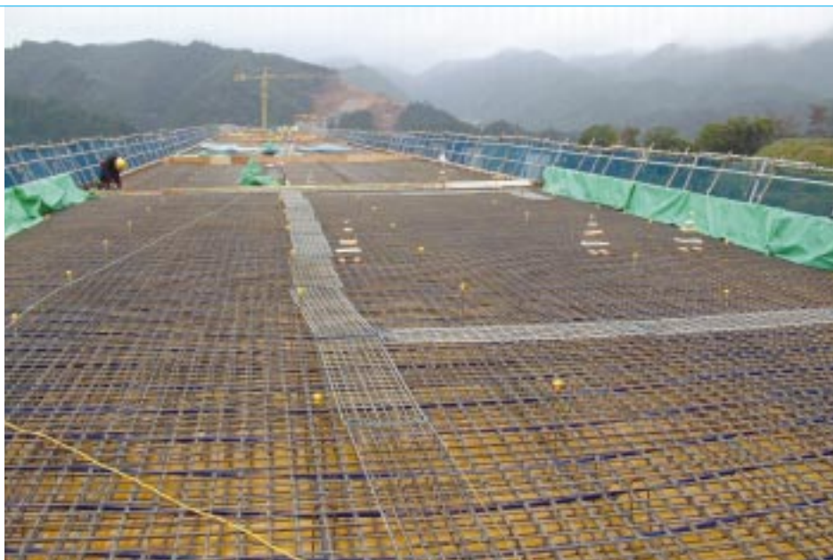
図1 PC床版 Prestressed concrete slab
