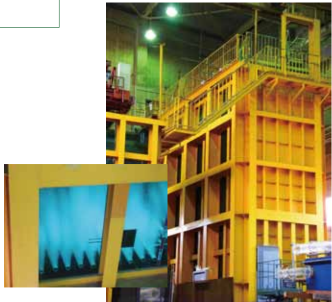
図9 深槽試験設備 Test facility
